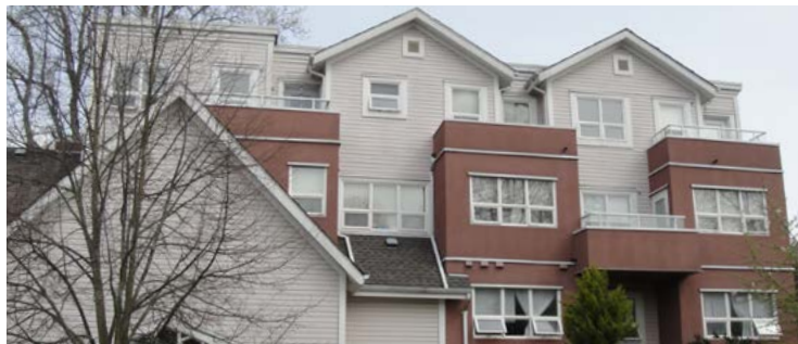
The CIP apartment units are located at St. George's Place.
